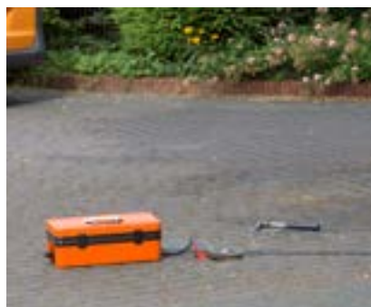
Acoustic location of main pipes
