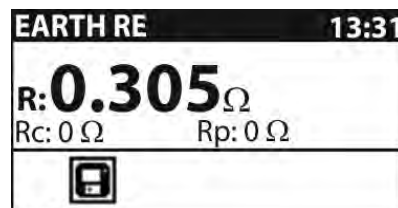
Fig. 26: Result screen of earth resistance measurement
