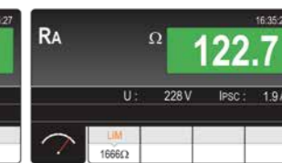
Measurement of overall earth resistance.
