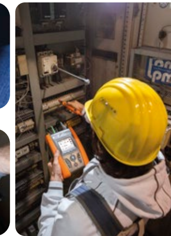
Start/stop measuring with remote lead PR400.
