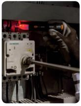
Step2 - Now rest and keep HT70 on the assumed phase L2 (on the conductor or sheath) for at least another 5s and wait for the LED to flash together with the buzzer sounding.
